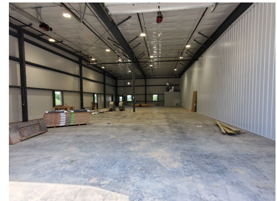
Warehouse Unit Heat Based on Warehouse Use & 200 Amp Electric Subpanel Provided by Landlord
